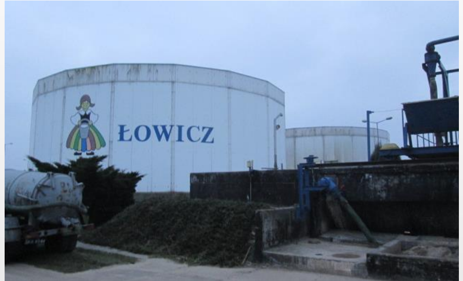
Dairy Factory, Poland, 2015
